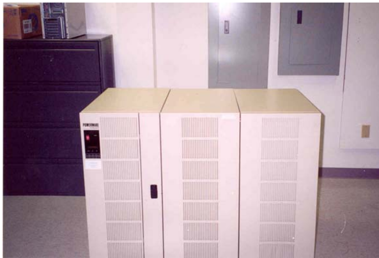
A PowerWare Plus UPS, capable of supplying power for 6 hours.
