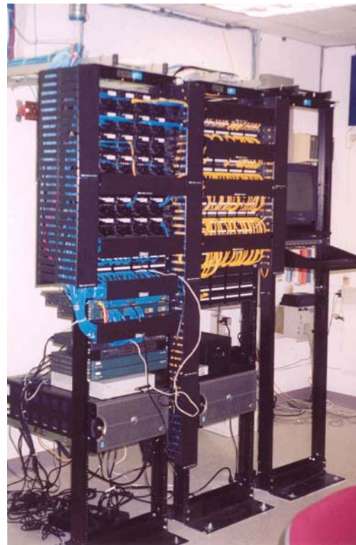
Oceania's Main Distribution Facility (MDF).
